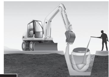
Water levels always in the primary and final chamber 200 mm higher than backfill
