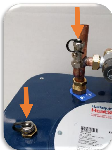
Figure 7 Filling loop connected
