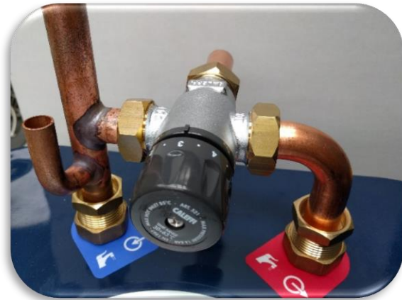
Figure 16 Mixer valve set to position #3
