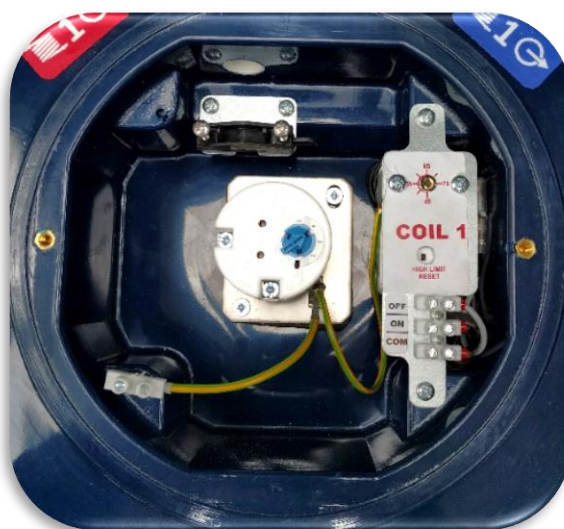
Figure 3 Top thermostat and immersion compartment
