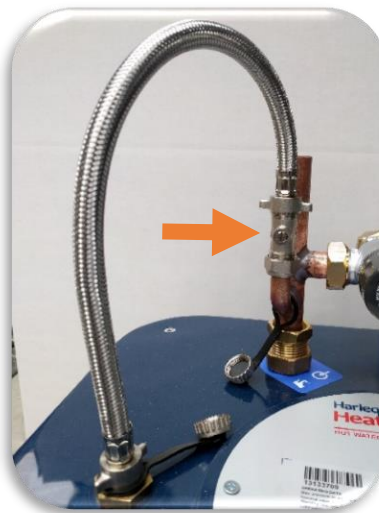
Figure 6 Filling loop disconnected
