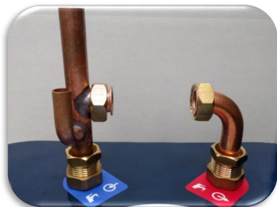
Figure 15 Mixer valve pipe set
