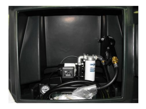
Image of 10 micron particle and water filter fitted to DS1300
