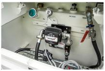
YARDMAX-FM-110V/240V: Electric fuel pump for dispensing diesel. Pump fitted with bypass, 1.2m suction hose, mechanical flow meter, 4m delivery hose & auto nozzle for safe refuelling.
